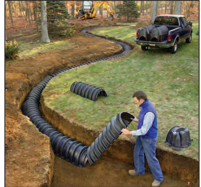
*Infiltrator chambers can be installed in curved, sloped and small areas allowing for optimal land use.*
